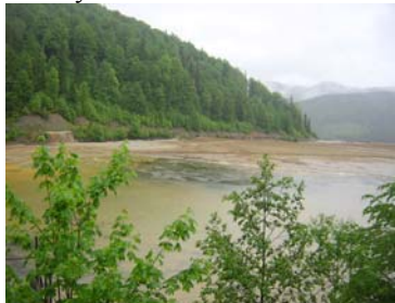
Figure 2 – The water screen from the beach of the decantation pool Valea Tărnicioara
