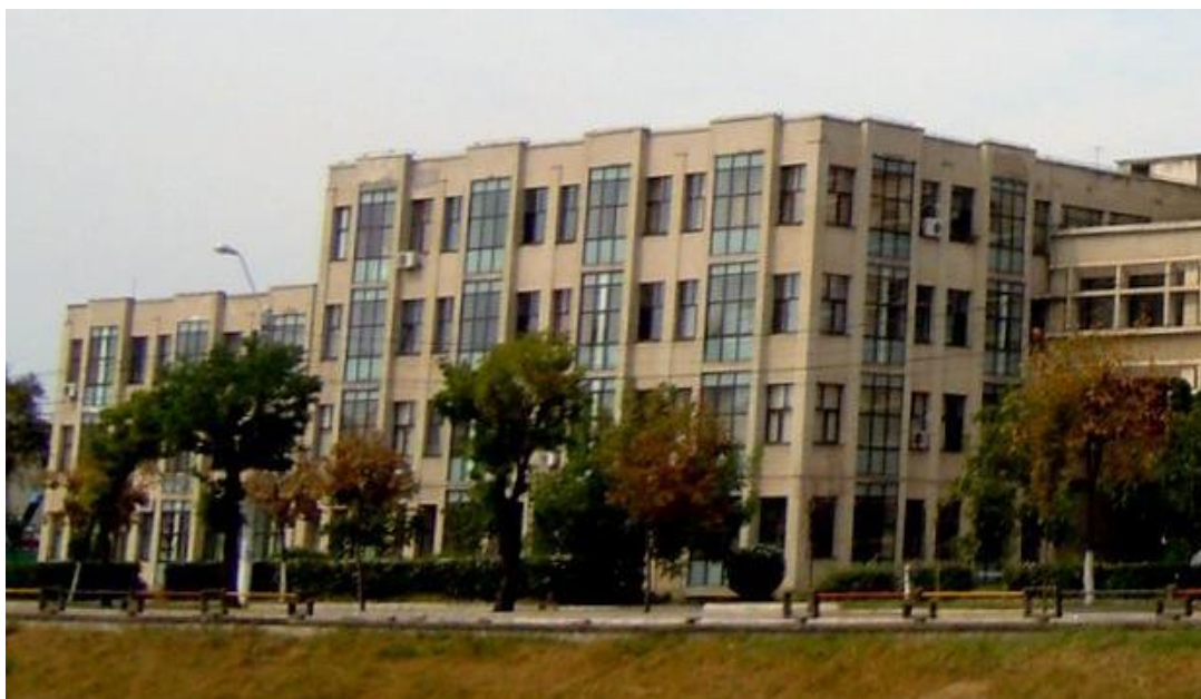
Figure 2. The Faculty of Electrical Engineering of Iasi.
